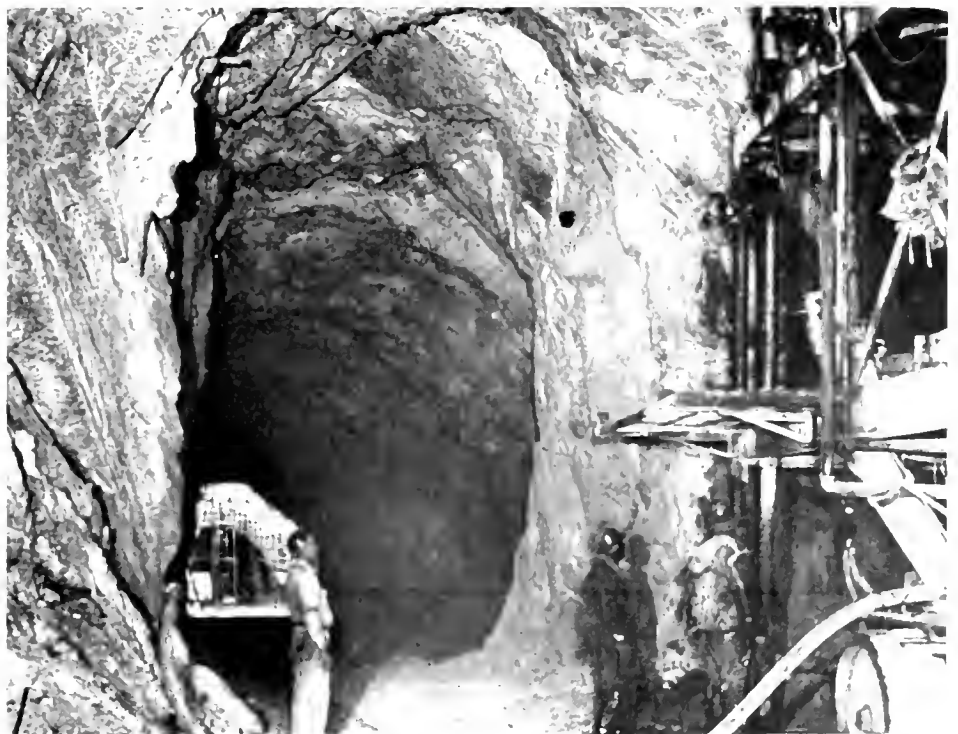
Equipment widening tunnel No. 1 bore. No. 2 bore entrance is seen in background
